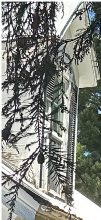
Figure 8: One intact shutter panel remains from original window shutters
