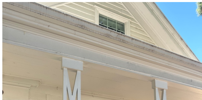
Figure 6: Ogee gutters above porch at front of house
