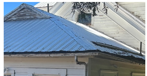
Figure 3: Decaying wood roof shingles covered with aluminum sheets, nailed down with board during last winter's storms
