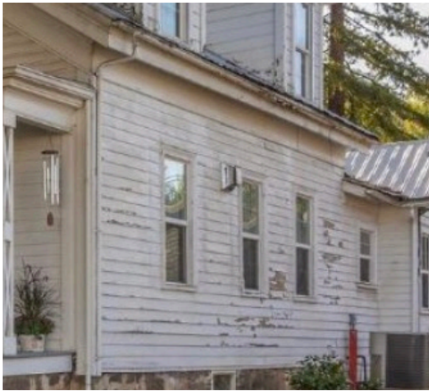
Figure 7: Peeling paint and decayed/rusted side gutters
