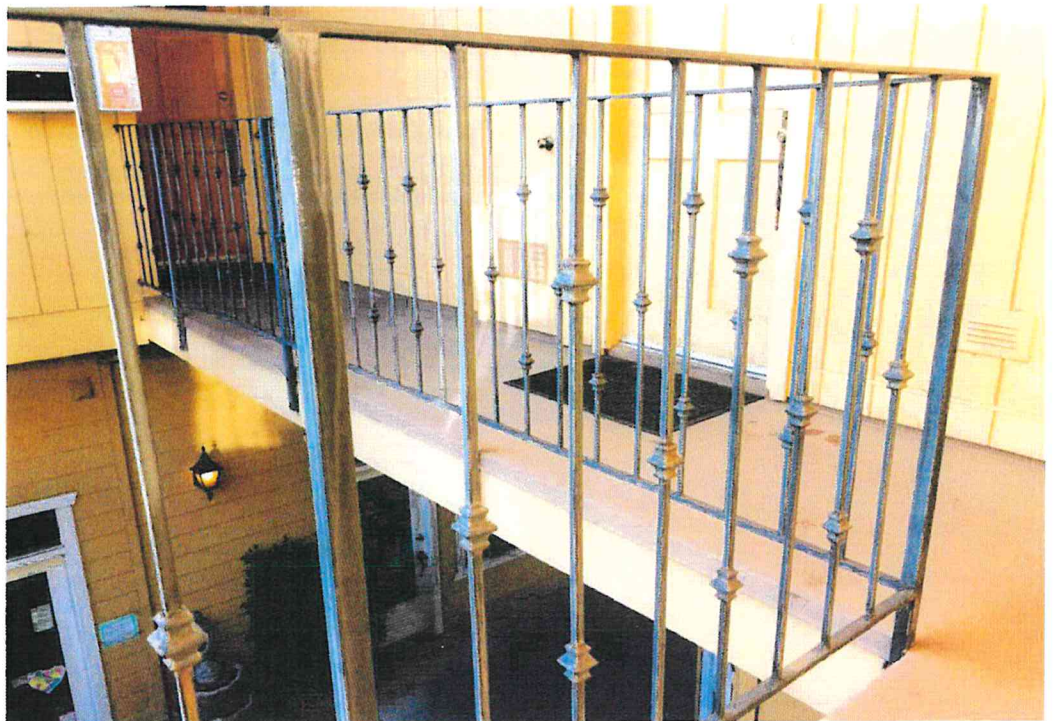
close up of railing upstairs. square tubing to be installed in between decorative knobs Spindles vertically and as needed
