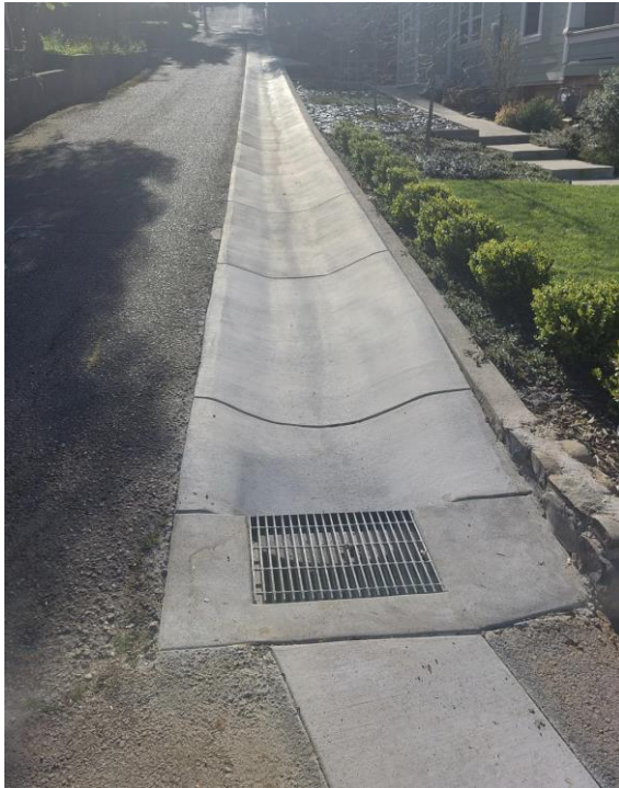
Worley storm drain ditch and new DI to street
